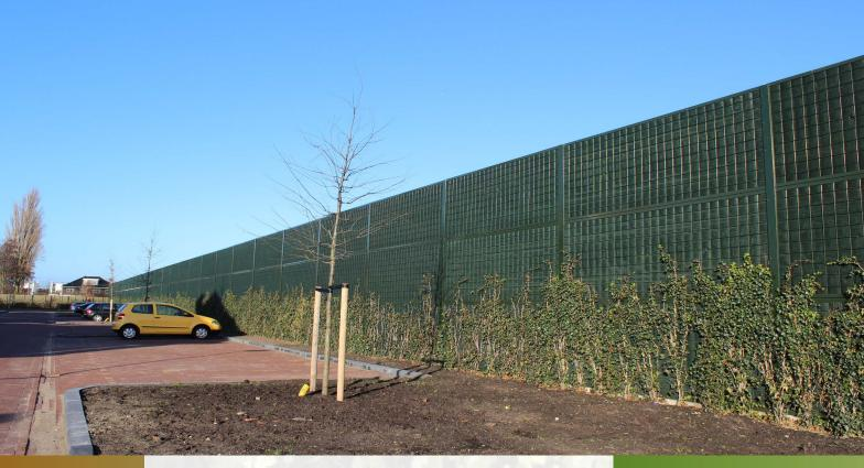
The Noise-Reducer® Noise Barrier is a lightweight construction with high insulation and absorption properties. On either the noise-side or on both sides of the panel, a galvanised steel wire-net and a polyethylene separator-net secures a layer of high absorptive mineral wool.
