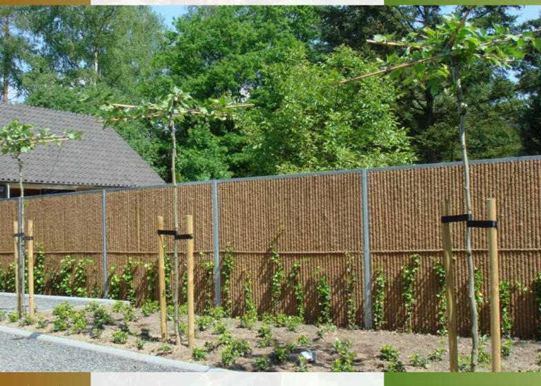
The **Kokowall**® Noise Barrier is a natural looking noise barrier system that befits any environment. The **Kokowall**® Noise Barrier panels finish consists of durable coconut fibre and is ideally suited for climbing plants. Coconut fibre has outstanding sound absorption properties. A **Kokowall**® screen will be covered in plants within a few years.
