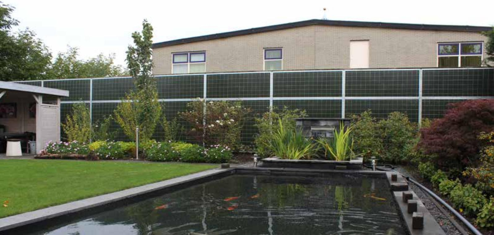
*The Noise-Reducer® Noise Barrier is a lightweight construction with high insulation and absorption properties. On either the noise-side or on both sides of the panel a galvanised steel wire-net and a polyethylene separator-net secures a layer of high absorptive mineral wool.*
